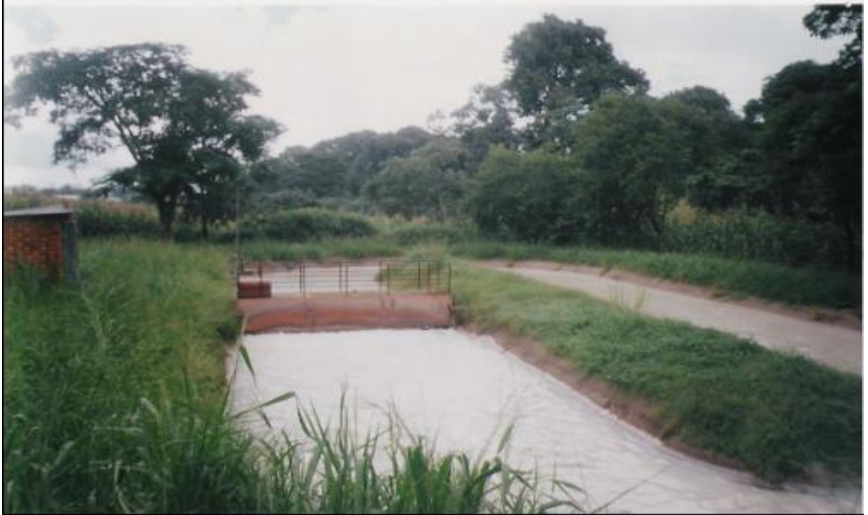
Figure 2.5: Oxidation ditch at dairy industry- Dairiboard
