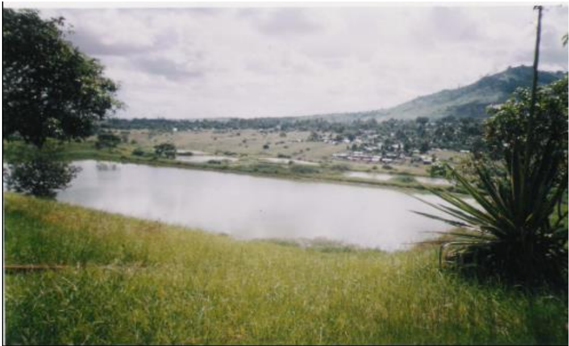
Figure 2.3: Limbe wastewater treatment plant showing pond system
