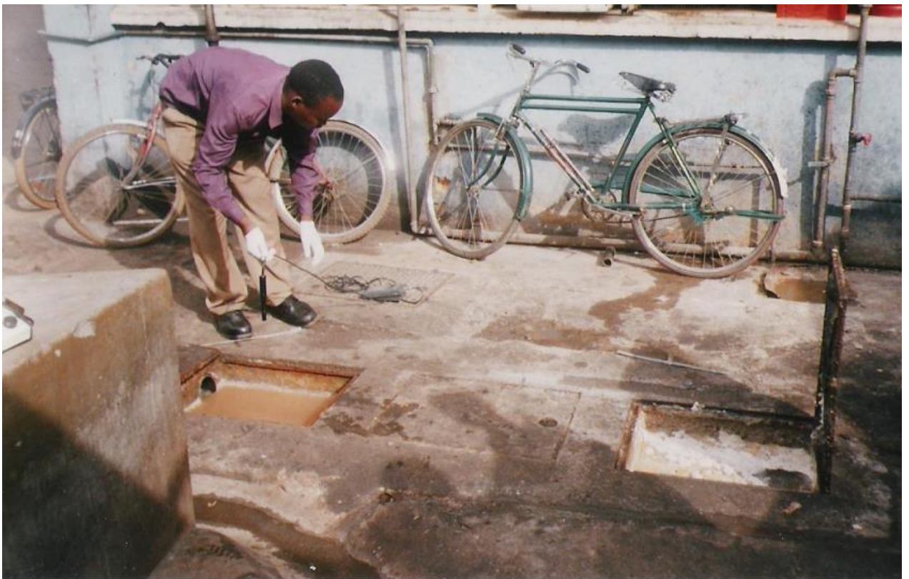
Figure 2.6: Oil interceptor at confectionery industry- Universal industries Ltd
